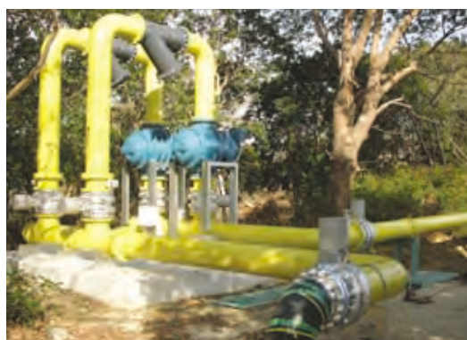
Piping for city gas receiving (Yokkaichi plant)
